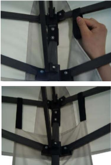
Fasten the leg textiles to the roof trusses using the Velcro fasteners.
